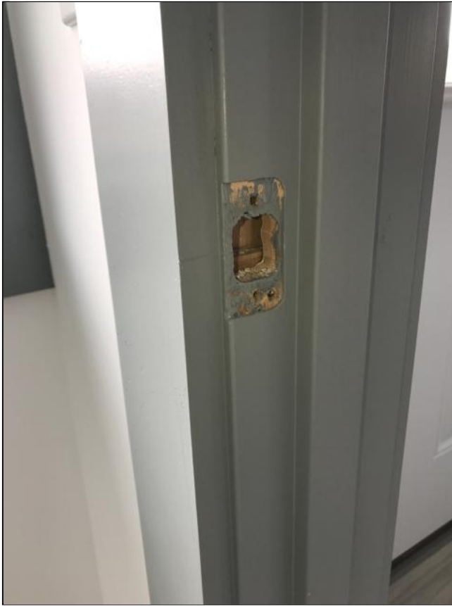
5.4 Item 1(Picture) Door slide/guide is missing in front office/bedroom
