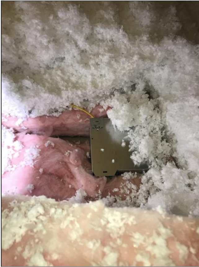
6.6 Item 1(Picture) Exhaust fan not venting to exterior
