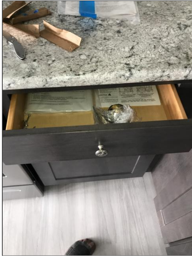
4.5 Item 2(Picture) Drawer does not soft-close as intended
