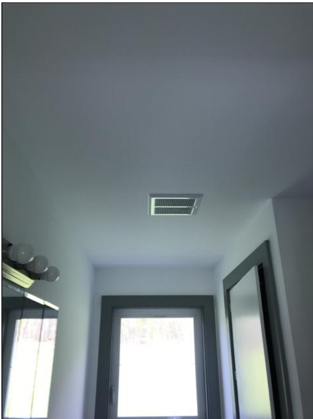
6.6 Item 3(Picture) Bath fan not venting to exterior
