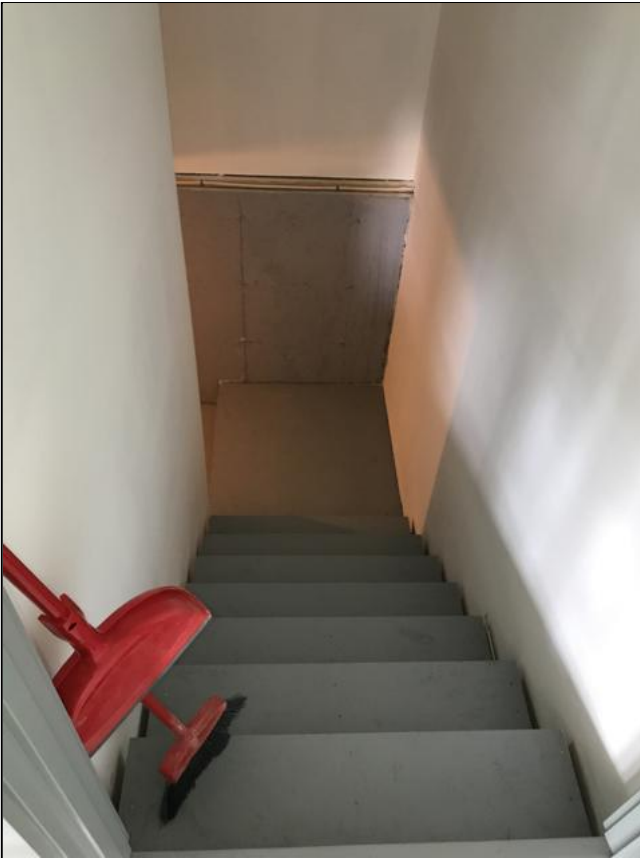
5.3 Item 1(Picture) Railing required on at least one side of stairs
