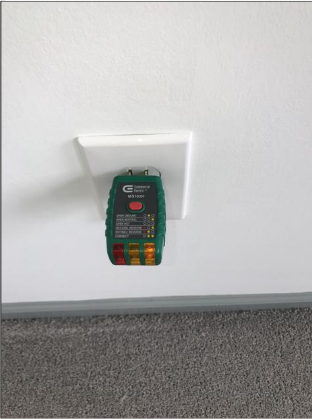
5.6 Item 1(Picture) Receptacle incorrectly installed
