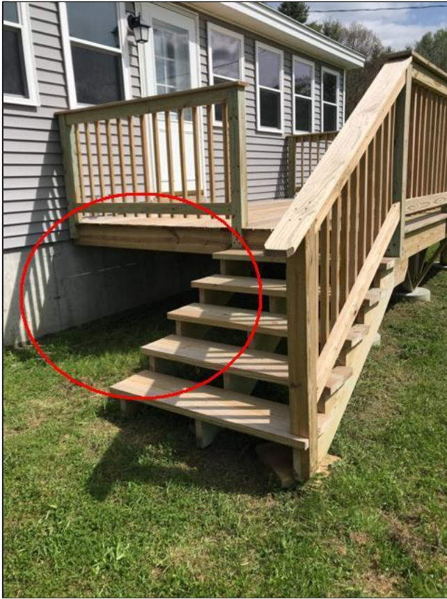
2.3 Item 1(Picture) Left side deck guard recommended
