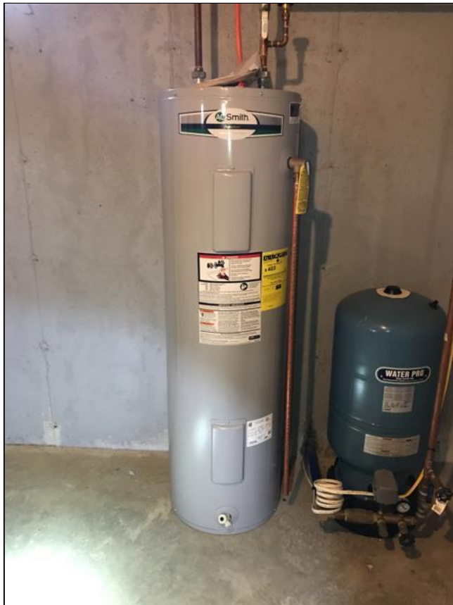
8.2 Item 1(Picture) Metal drain pain recommended beneath water heater
