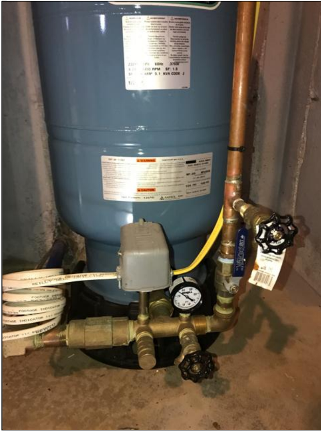
8.1 Item 1(Picture) Well pressure tank
