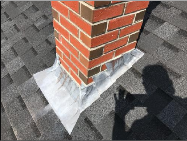
1.2 Item 3(Picture) Lead flashing around chimney
