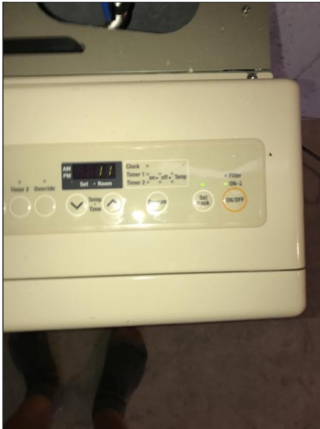
10.0 Item 1(Picture) Error code 11 on each heater
