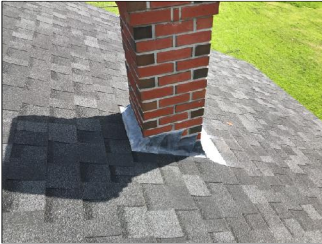
1.2 Item 1(Picture) Lead flashing around chimney
