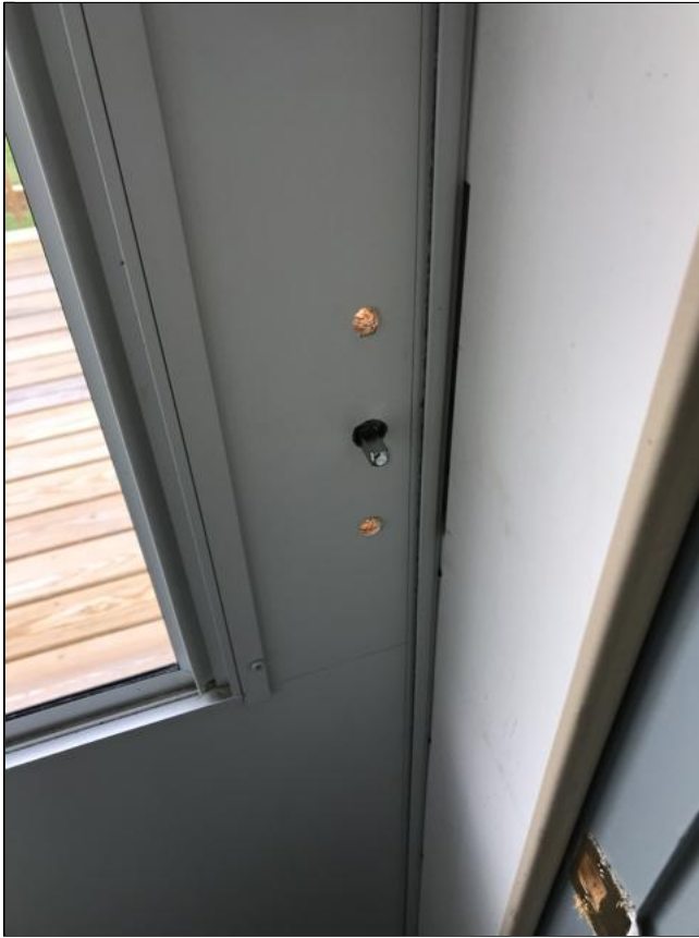
2.1 Item 1(Picture) Door to deck is missing doorknob to enter/exit
