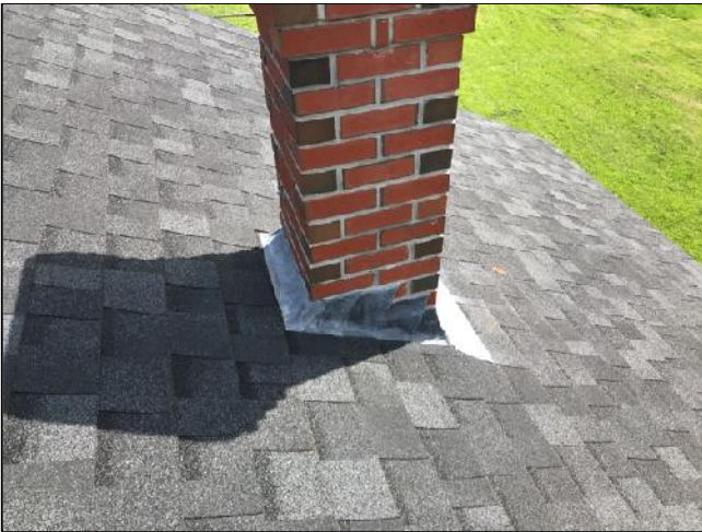
1.2 Item 1(Picture) Lead flashing around chimney
