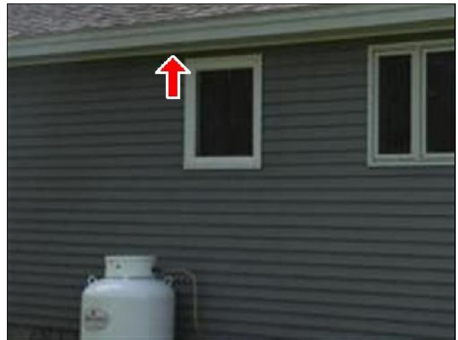
6.6 Item 4(Picture) Bath vent to exit soffit
