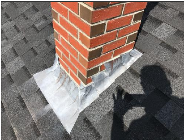
1.2 Item 3(Picture) Lead flashing around chimney
