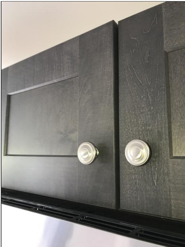
4.5 Item 3(Picture) Door does not close flush
