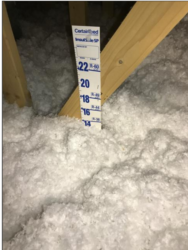
1.7 Item 2(Picture) 14-16" of insulation in attic
