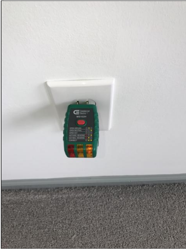
5.6 Item 1(Picture) Receptacle incorrectly installed
