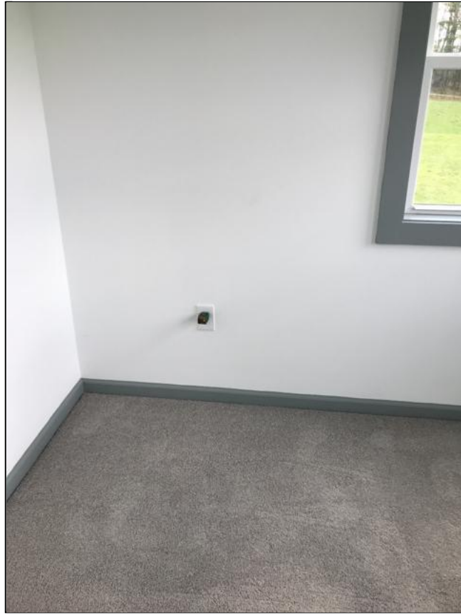
5.6 Item 2(Picture) Receptacle incorrectly installed
