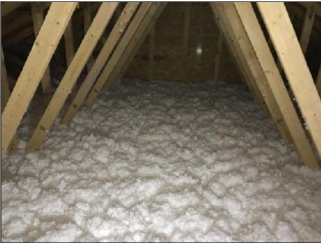
1.7 Item 1(Picture) Insulation in attic
