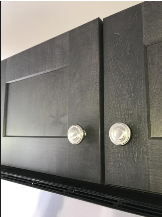
4.5 Item 3(Picture) Door does not close flush
