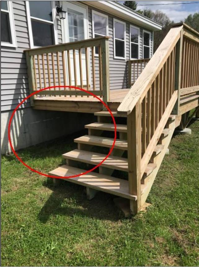
2.3 Item 1(Picture) Left side deck guard recommended
