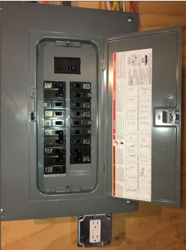
9.1 Item 1(Picture) 100 amp panel in basement
