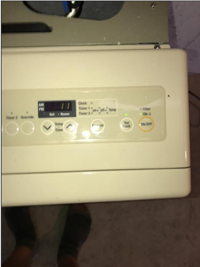
10.0 Item 1(Picture) Error code 11 on each heater
