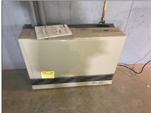
10.0 Item 2(Picture) Rinnai heater in basement and 1st floor
